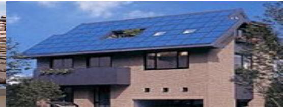
Solar Roof Modules
